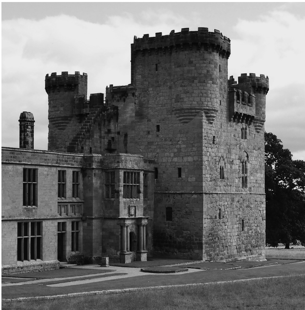
Belsay: Tower house from the SW.
